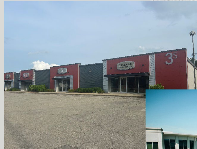
Schmoll Industrial Park, Indianapolis, IN
