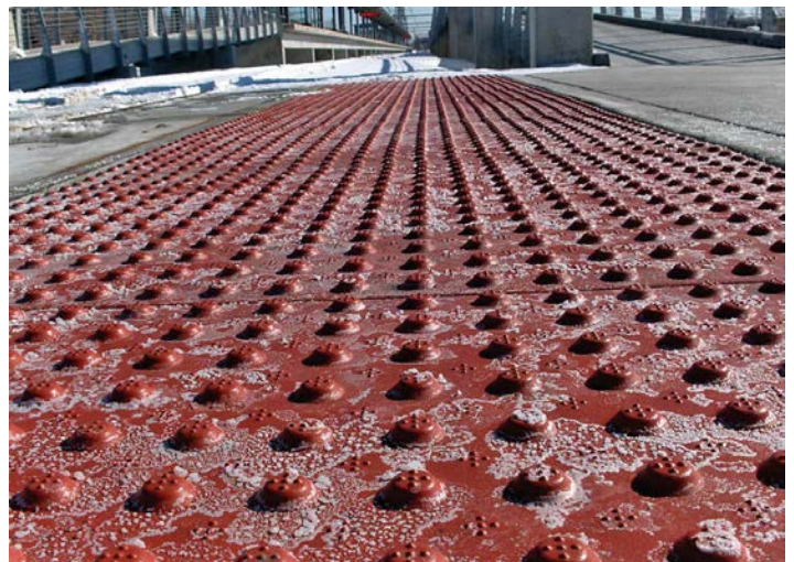
Detectable warnings come in a variety of styles, colors, and materials including brick or concrete unit pavers (left) and steel plates (right).
