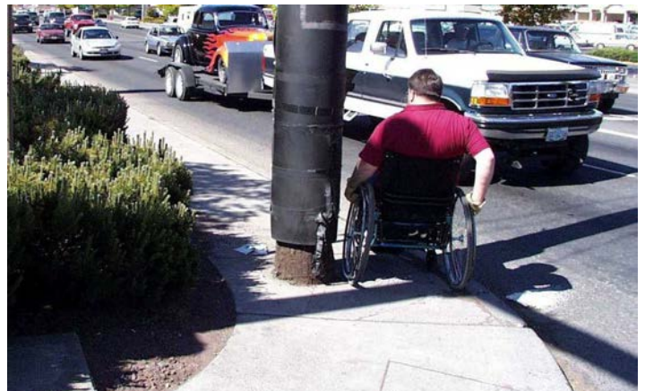
Obstructions in the sidewalk can create access issues for wheelchairs and other vulnerable users.
