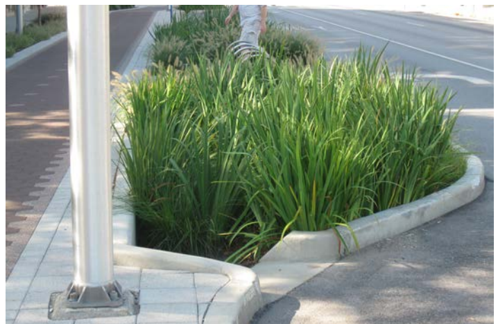
Rain gardens, also known as stormwater planters, such as those pictured above can be used to slow stormwater runoff and filter the first flush of pollutants as they run off the roadway. When combined with other ornamental plantings they can contribute to overall downtown aesthetics.
