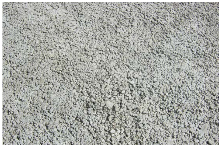
The alley pictured at top and detailed above looks very similar to traditional concrete. In reality it is porous pavement that allows stormwater to run though it and infiltrate the ground. It does require annual maintenance vacuuming to ensure the pores do not fill with sediment.
