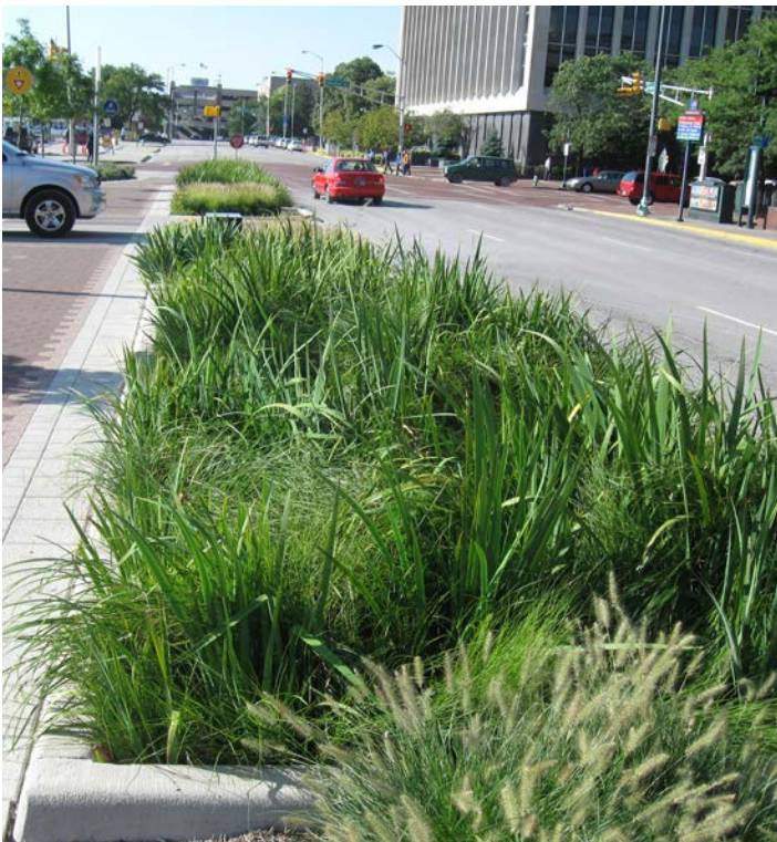
A bioretention facility used to filter stormwater and increase infiltration.
