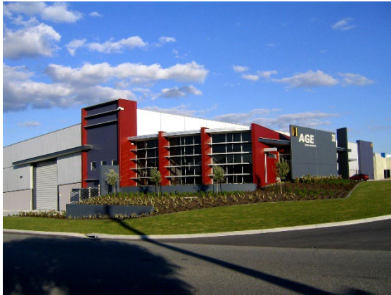
Figure 3: Ag Sciences Industrial Building
