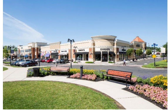
Figure 12: Shops at Valley Square, Warrington, PA
