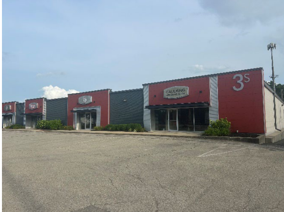
Figure 3: Schmolz Industrial Park, Indianapolis, IN
