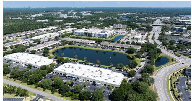
Figure 2: Gateway Park, Jacksonville, FL
