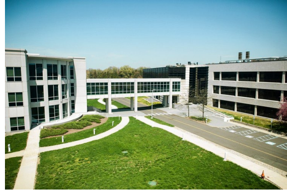
Figure 6: NJ Center of Excellence, Bridgewater, NJ
